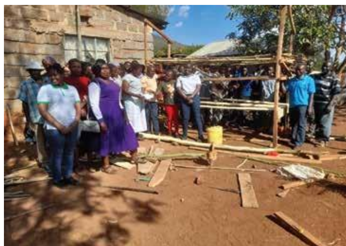
Demonstration of construction of an improved poultry house
